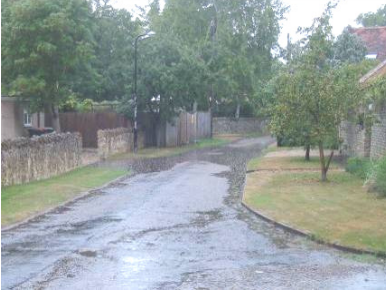
Minor flooding of road
