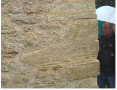
Oolitic limestone and shelly limestone with cross-bedding, outer wall of St Peters Church
